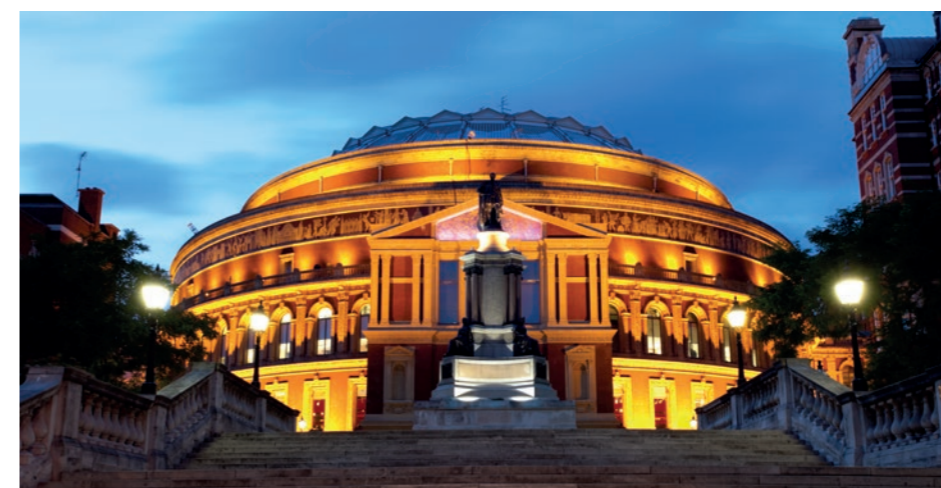
The Royal Albert Hall, London, UK An Advanced fire system protects this iconic Grade I-listed concert hall, opened by Queen Victoria in 1871.
