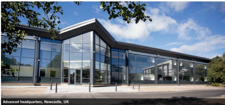
Advanced headquarters, Newcastle, UK
