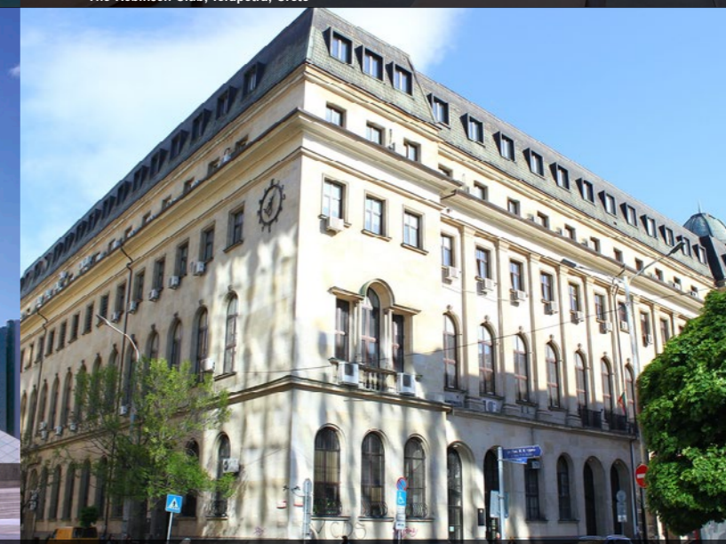
Communications Regulation Commission office, Sofia, Bulgaria
