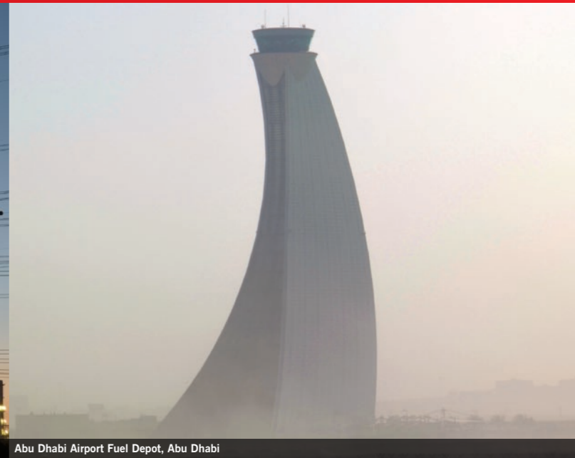
Abu Dhabi Airport Fuel Depot, Abu Dhabi
