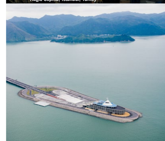
Macau Bridge, Hong Kong, China
